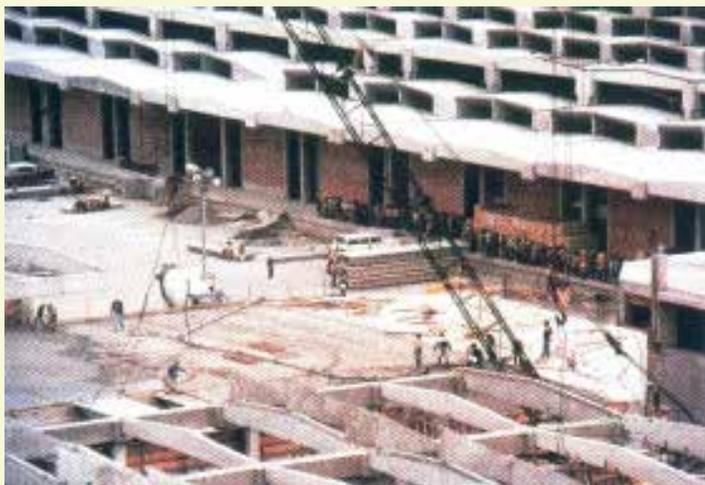
In January, 1982 the progress of the work showed 3 thousand and 5 hundred people working. The foundation was achieved through an excavation of 399 thousand and 692 square meters, using 17,000 tons of steel, 86 thousand square meters of concrete, 77 thousand square meters of slab lid and 14,000 meters of drainage pipe.
